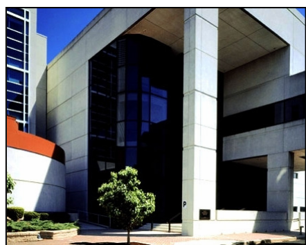
Picture caption: Vetter's Chicago facility at the Illinois Science + Technology Park.
