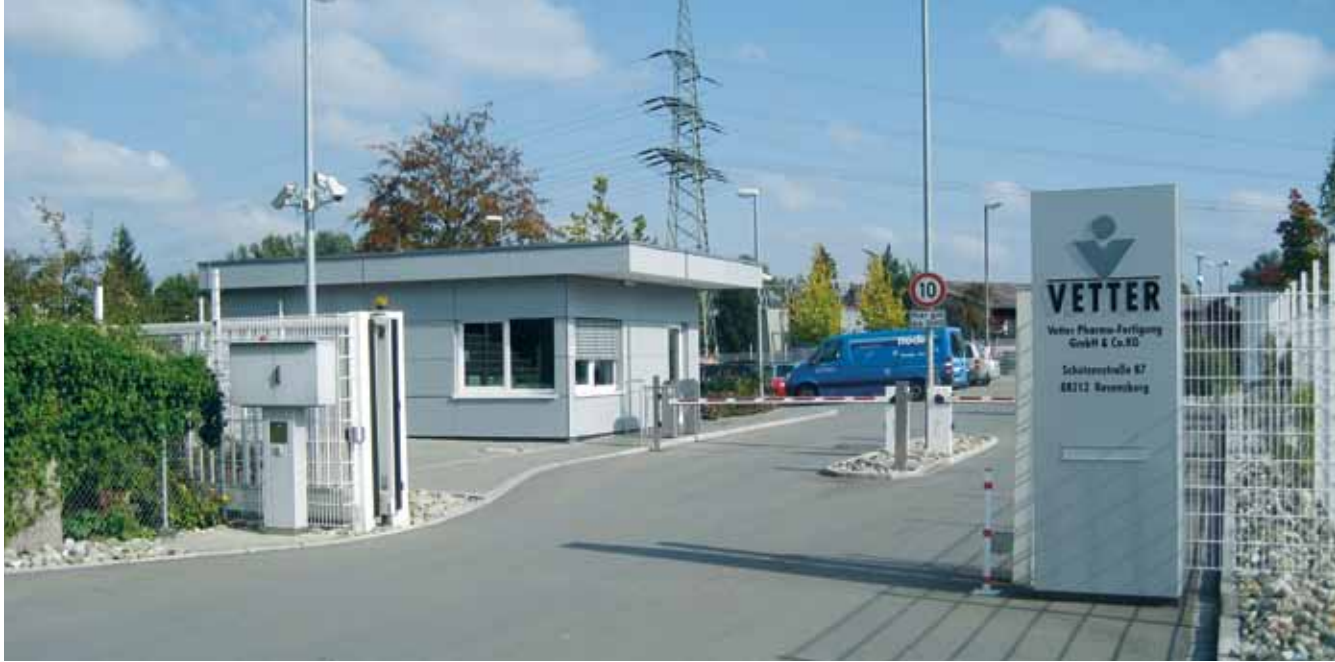
Access road to the Schuetzenstrasse building with a gate and barrier system.
